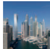
DUBAI Saving energy in air conditioning systems
